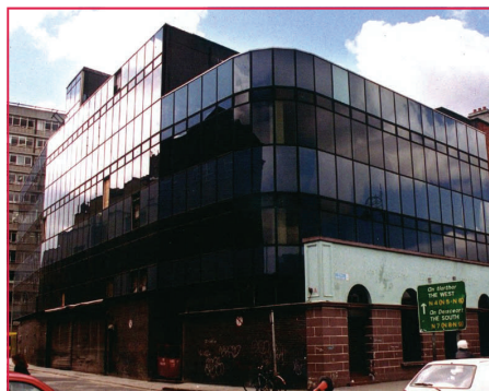
Burgh Quay before reconstruction
